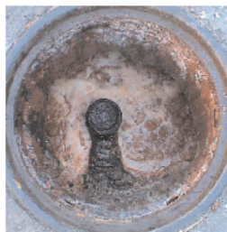
Prior to Treatment
